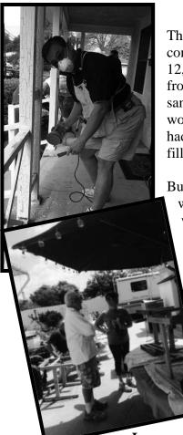
The **South Bay Sunrise Rotary Club** converged on Southwest House on April 12, 2014, and spent the day fixing up the front porch. The front trim was scraped, sanded, primed and painted. Some of the wood was in such poor condition that it had to be replaced, while some of it needed filling with putty.
